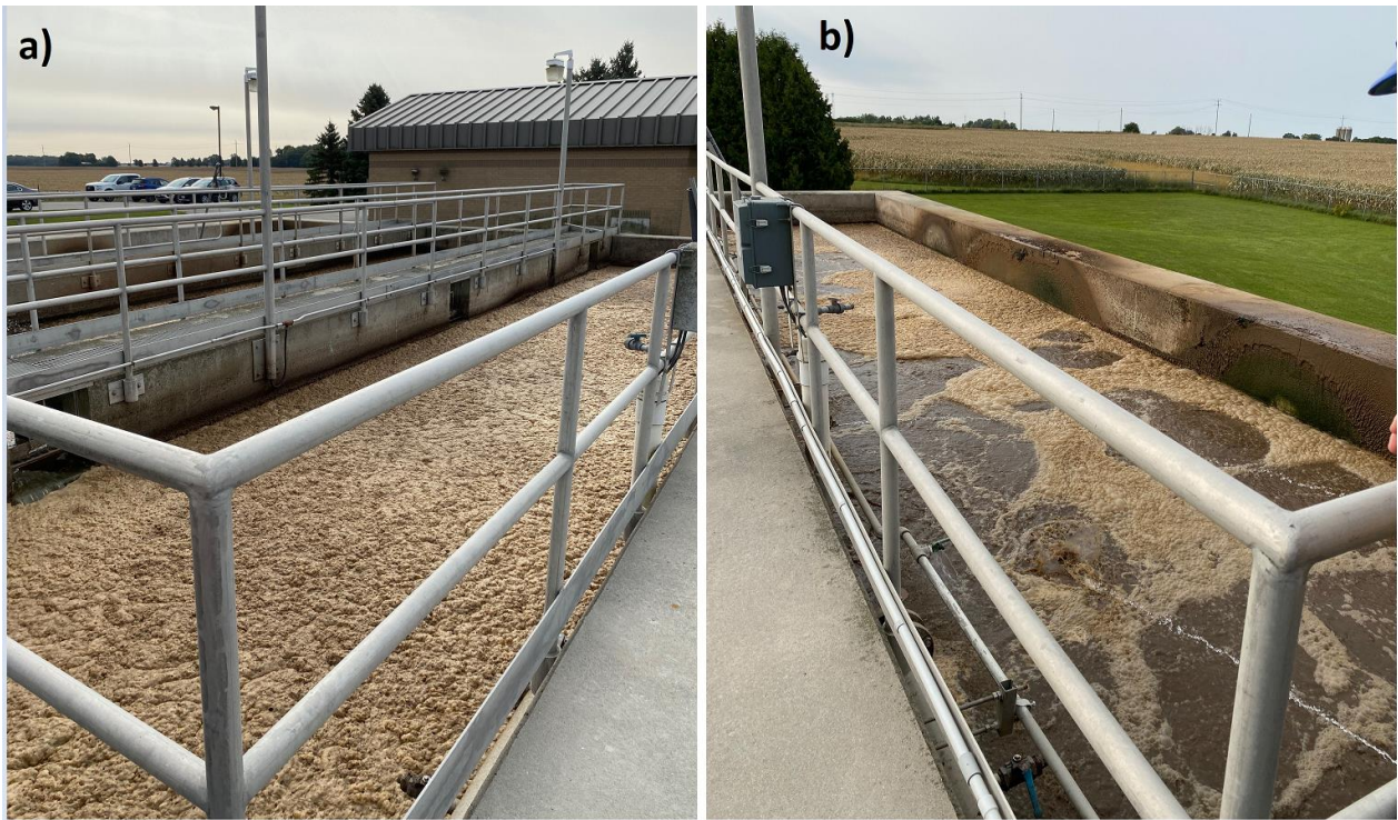
Figure 1 – Foam on the Surface of the Bioreactors in a) Pass 1 and b) Pass 2
