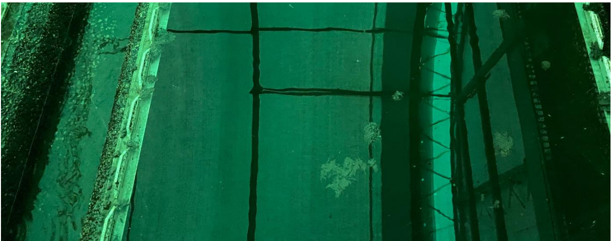
Figure 4 – Example of Rising Sludge Observed in Secondary Clarifiers
